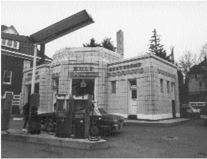
Transportation concerns pervade the history of Bedford, Pennsylvania. The Bedford Historic District includes this ca. 1936 Art Deco gasoline station for its association with early automobile travel on the Lincoln Highway (present-day Route 30). Photo by Tanya M. Velt.
