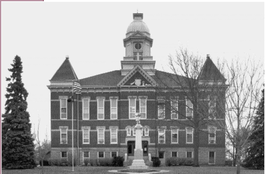
Communities across the country include districts, sites, buildings, structures, and objects listed in the National Register of Historic Places. Historic courthouses, like the Washington County Courthouse in Blair, NE, represent the heritage of older communities. Photo by B. R. Long. Four
