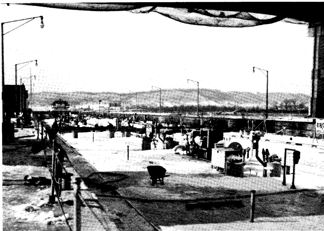
Towboat and petroleum barges lodged in Markland Locks during the February 1978 ice jam. Visible at the top is Markland Bridge then under construction with safety nets suspended below it.
