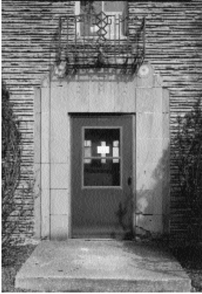
The door surround on the Wieboldt-Rostone House (Walter Scholer, 1933) is the only area of the exterior where the original building material, Rostone, a precast form of simulated masonry, is intact.
