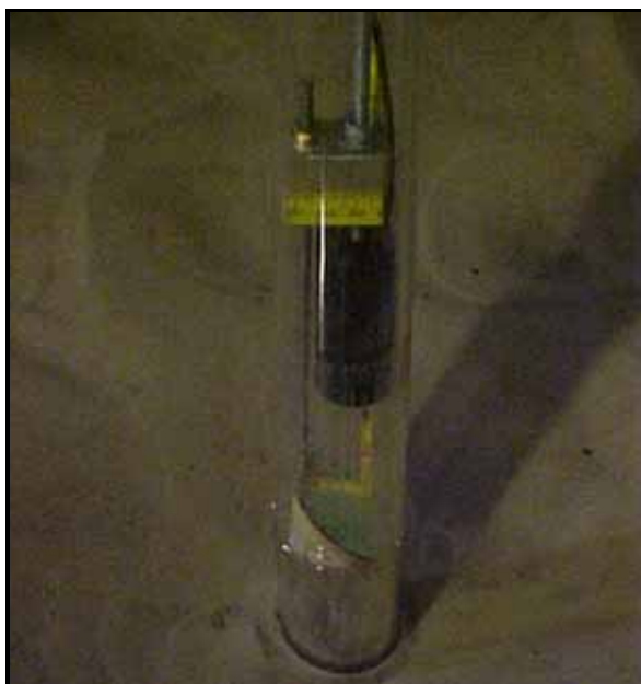
Figure 19. Camera-mirror system installed inside the pier.
