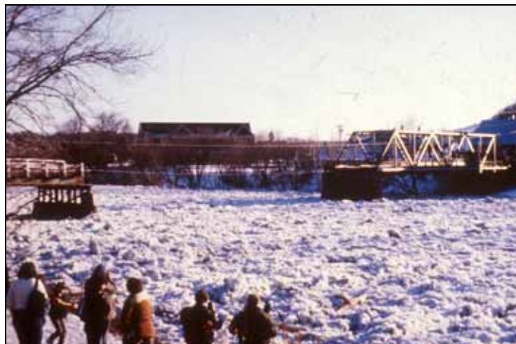
Figure 2. Failure of the Bridge Street Bridge, 26 January 1990, looking downstream.
