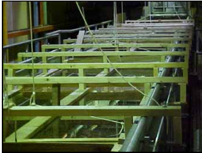
Figure 14. Ice restraint system upstream.
