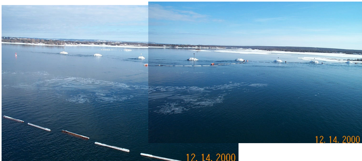
Figure 4. Completed ice stabilization islands and east arm of ice boom, December 2000.
