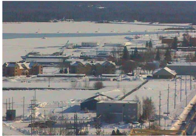
Figure 22. 20 January 2000. By this date, an ice arch had formed upstream of the Little Rapids Cut.
