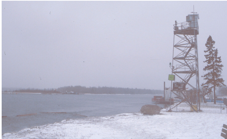
Figure 7. Tower at Mission Point, site of second Webcam and U.S. Coast Guard video camera. The west arm of the boom is on the left and the Sugar Island Ferry slip appears in the background.
