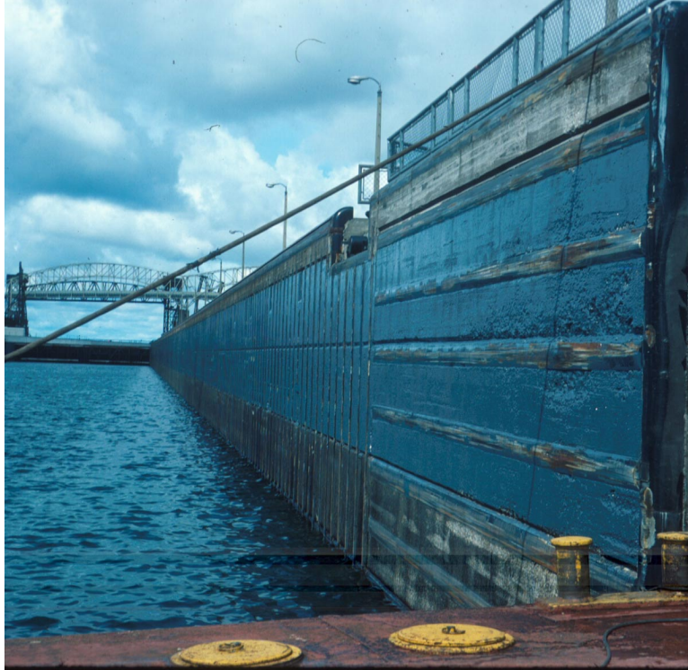
Figure 8. Copolymer coating at the Soo Locks.
