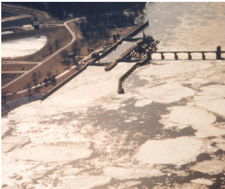
Figure 3. Ice accumulation in the upper approach at Lock and Dam 21 on the upper Mississippi River.
