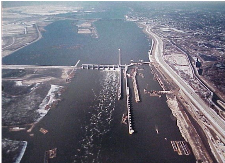
Figure 4. Mel Price Lock and Dam on the Mississippi River at Alton, Illinois.
