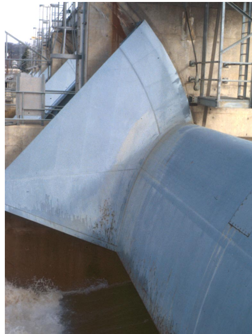
Figure 20. Submergible gate at Marseilles Dam.
