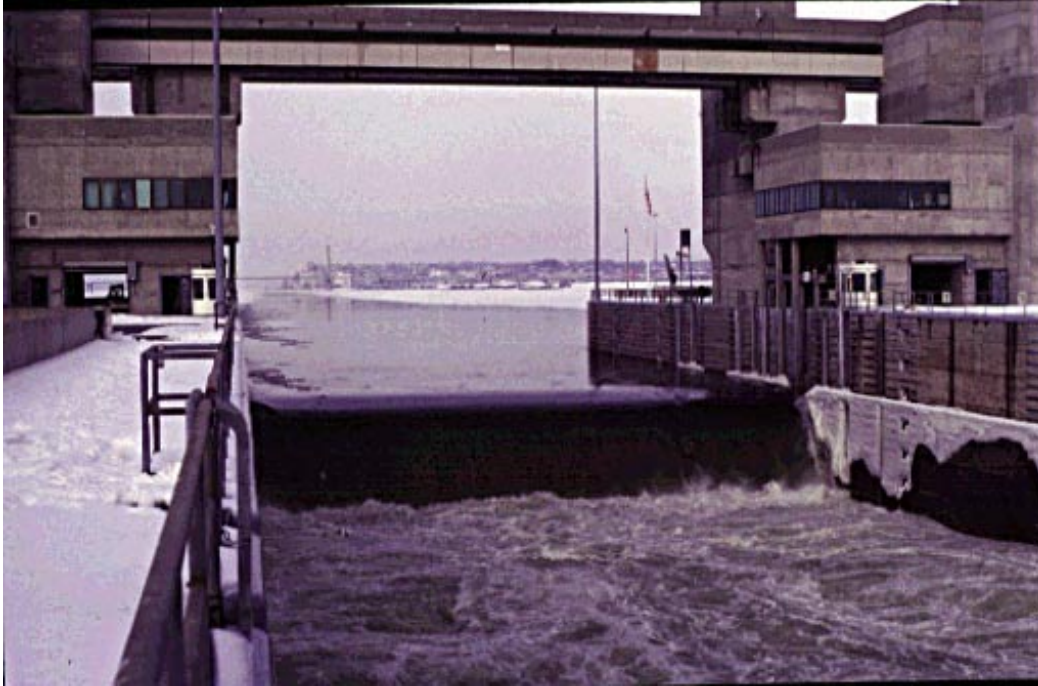
Figure 12. Submersible lift gate at Mel Price Lock.
