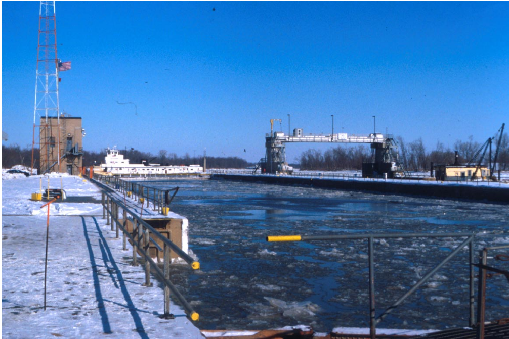
Figure 14. Le Grange Lock and Dam on the Illinois River. A free towboat washes brash ice from the upper approach, towards the submergible gate, adjacent to the lock chamber.
