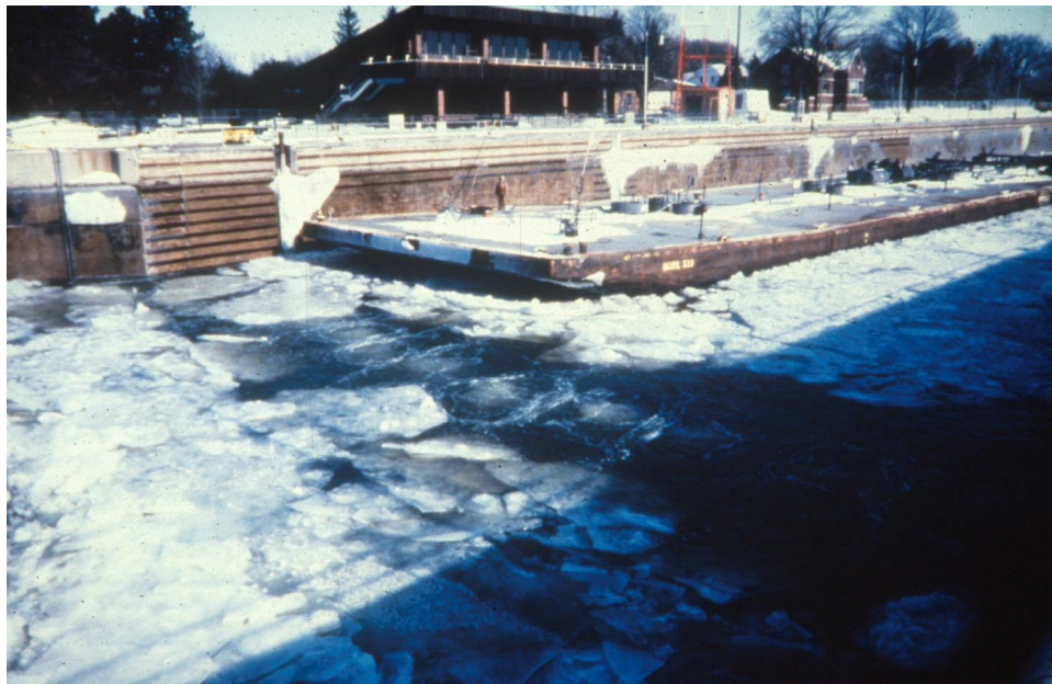
Figure 18. Lower sill curtain at Starved Rock Lock.
