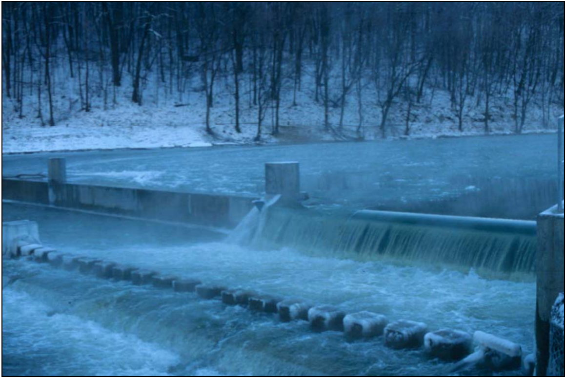
Figure 3. Frazil slush accumulating behind the Oil Creek ice control weir, Oil City, Pennsylvania.
