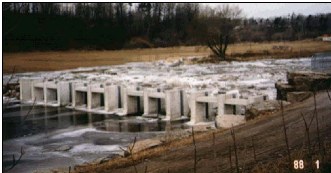
Figure 5. Credit River pier ice control structure, Mississauga, Ontario.
