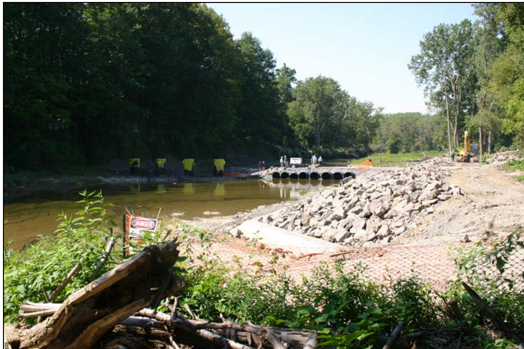
b. ICS under construction, summer 2005.
