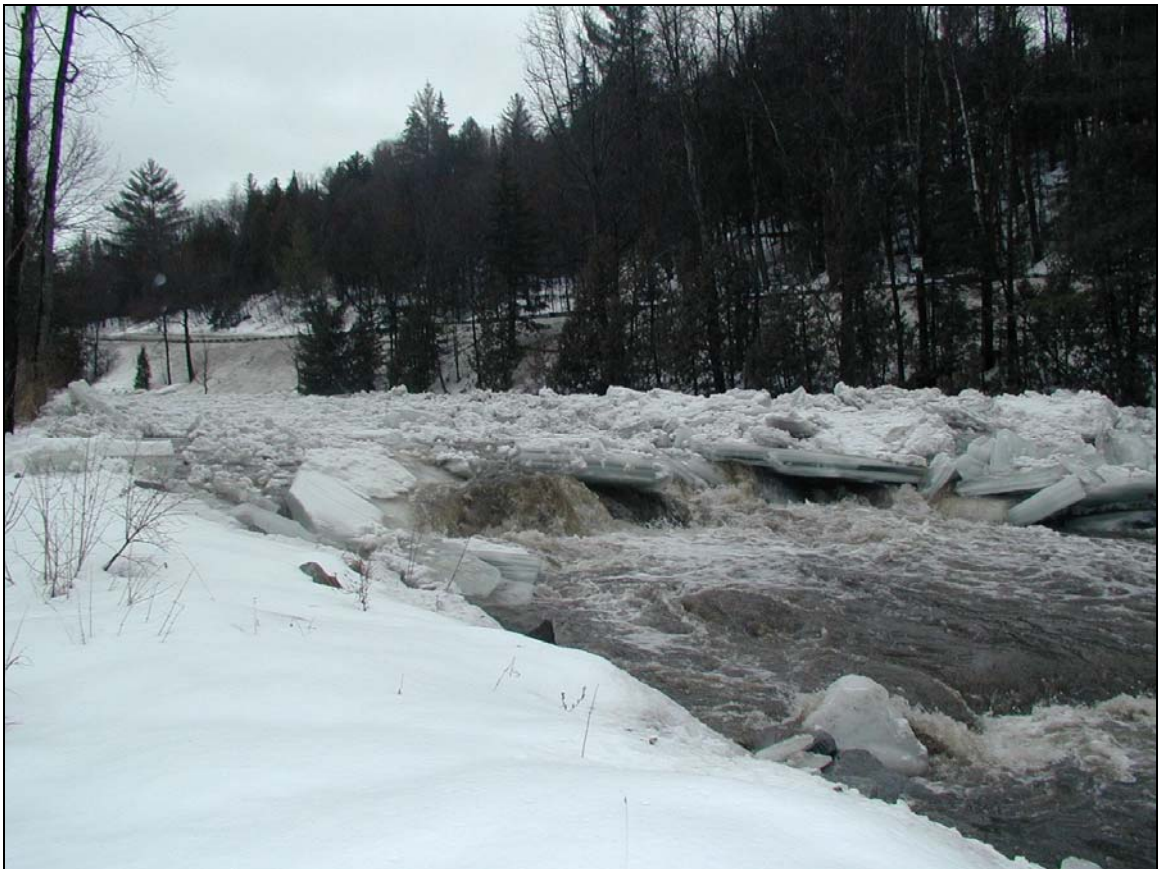
Figure 6. Ice jam at the granite block ice control structure on the Lamoille River upstream of Hardwick, Vermont.
