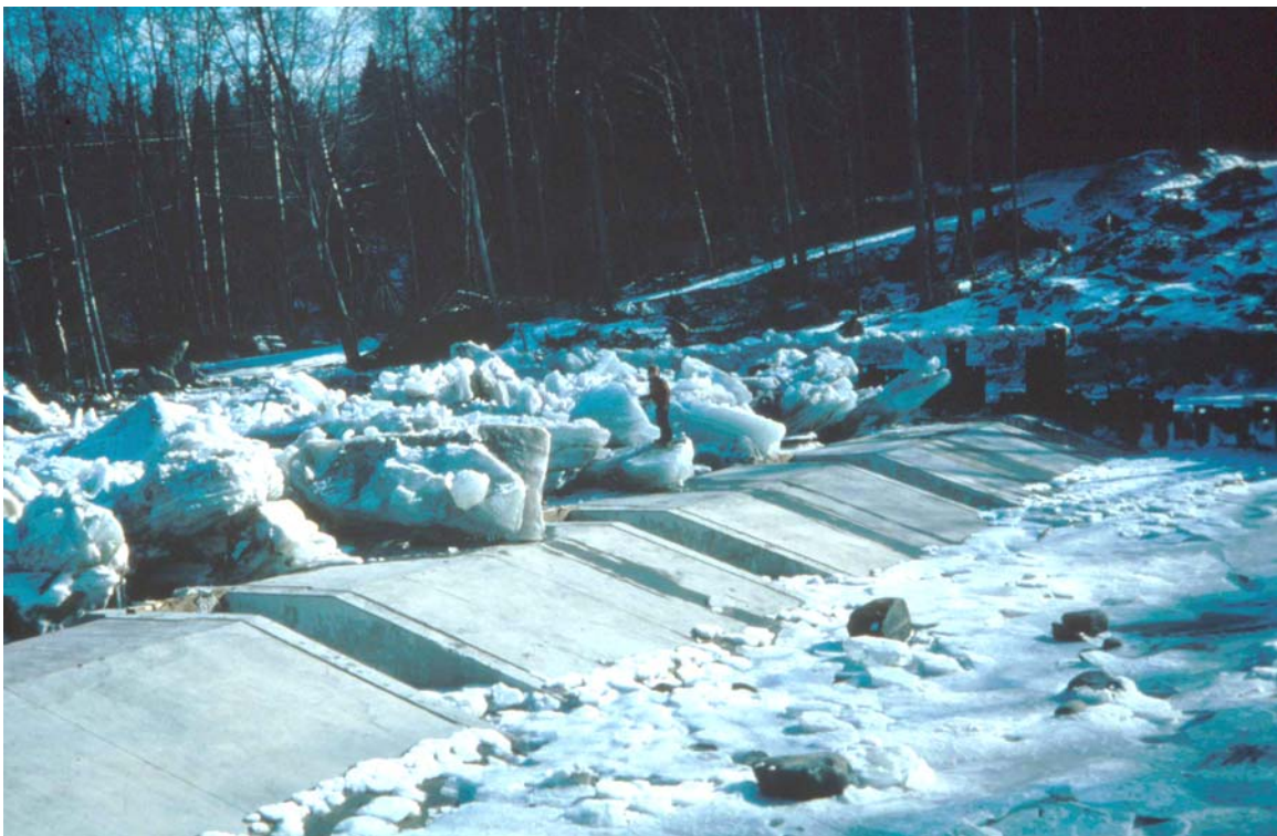
Figure 1. Breakup ice run retained by frazil ice retention weir on the Israel River upstream of Lancaster, New Hampshire.
