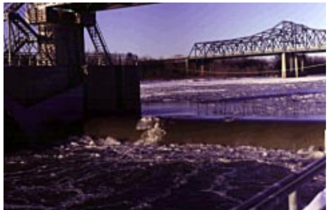
Figure 9. Submergible gate at Peoria Lock and Dam on the Illinois Waterway.
