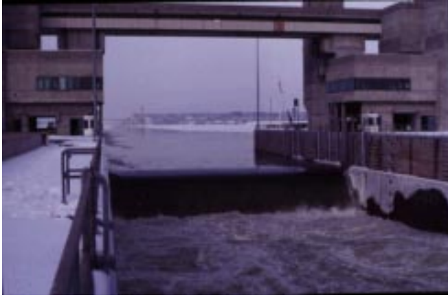
Figure 8. Passing ice over the upstream lift gate of the main lock at Melvin Price Lock and Dam on the Mississippi River.
