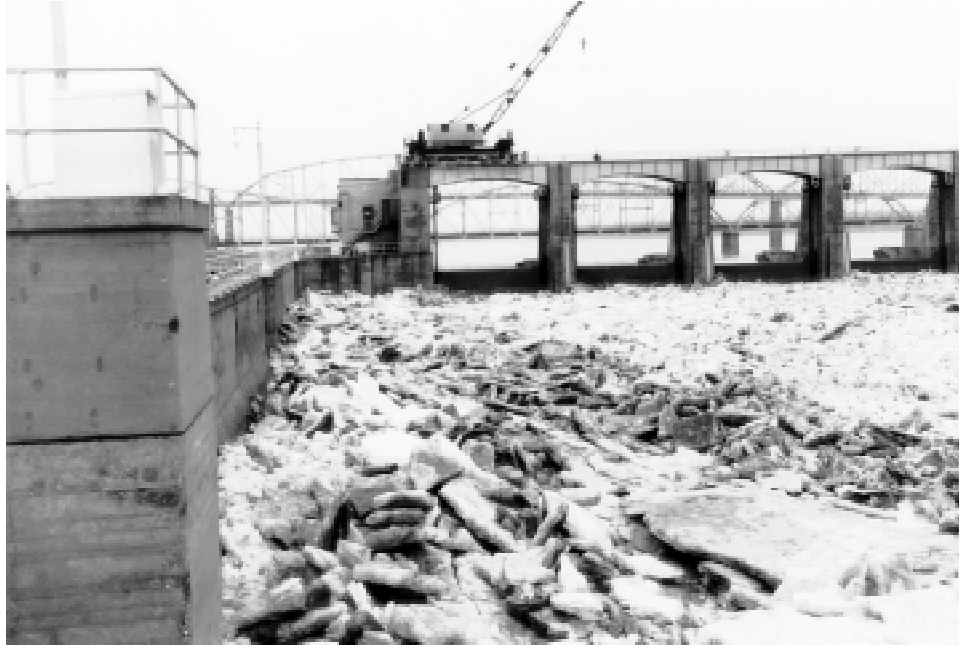
Figure 7. Accumulation of broken ice upstream of Lock and Dam 26, 11 February 1966, Alton, Illinois.
