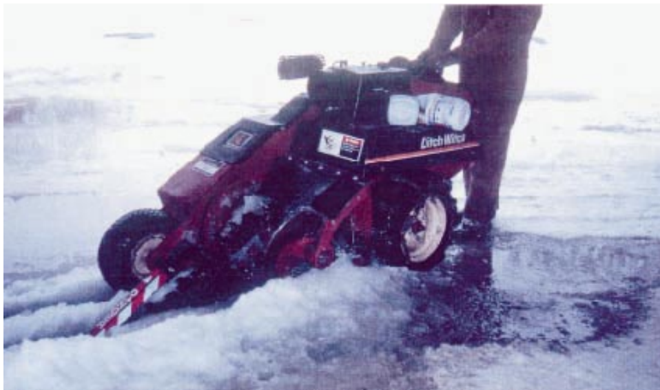
b. Ditchwitch 1260 cutting ice in Montpelier, Vermont.
