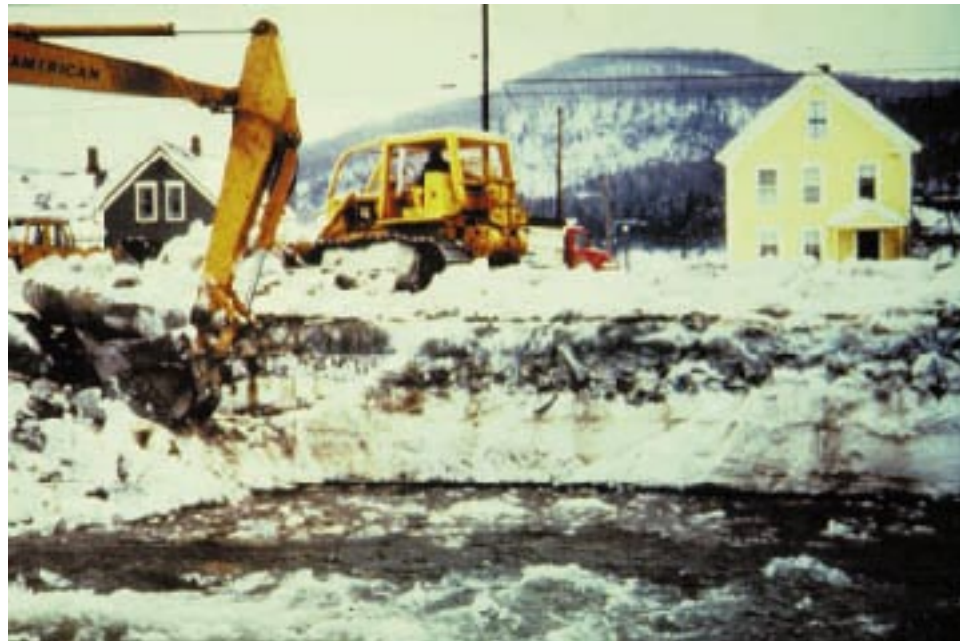
Figure 19. Breaching an ice jam in Hardwick, Vermont, using excavation equipment working from the shore and a bridge (bridge is not shown, but is just beyond the left edge of the photograph).
