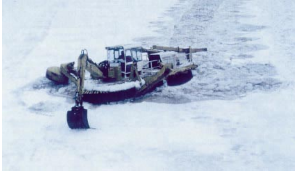
Figure 12. Breaking ice with an amphibious excavator on the Aroostook River, Ft. Fairfield, Maine.
