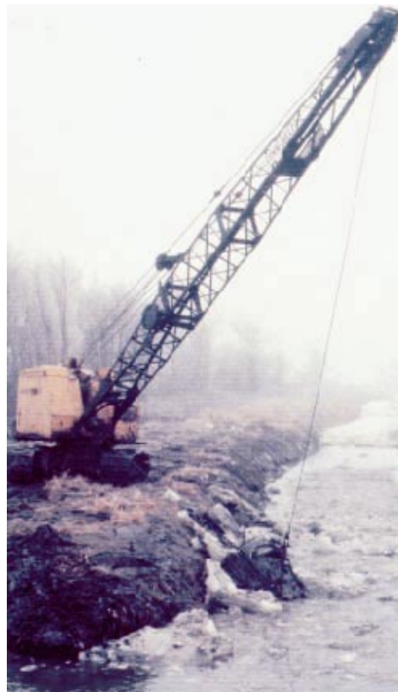
Figure 11. Using a bucket dredge to break ice in a river.
