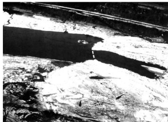
Figure 4. Parallel ice shear walls at the Allegheny River ice boom.
