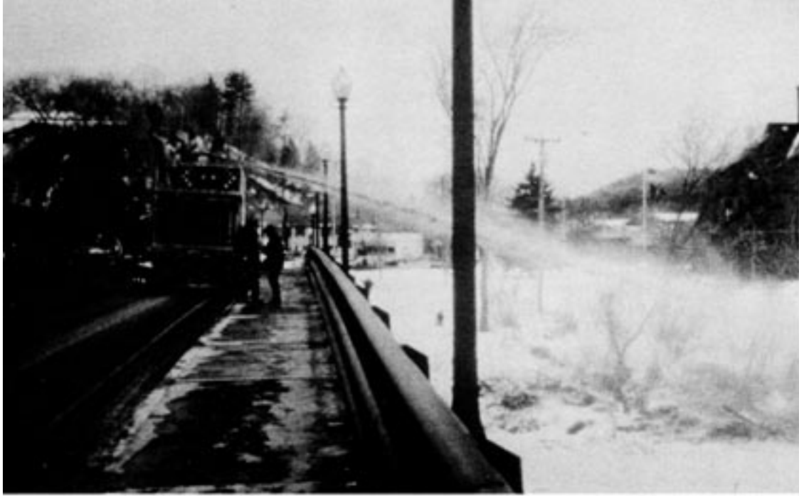
Figure 11. Hydroseeder being used to put leaves on the White River in Hartford, Vermont (March 1994).
