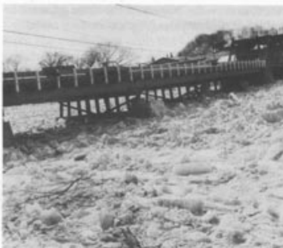
Figure 4. Temporary piers subjected to ice forces in 1969.
