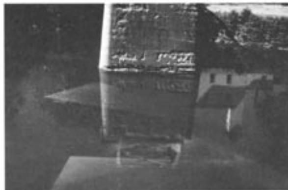
Figure 6. Piers on the river bottom.
