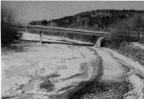
Figure 7. Route 5 bridge, February 1992, showing ice conditions upstream of the instrumented bridge.
