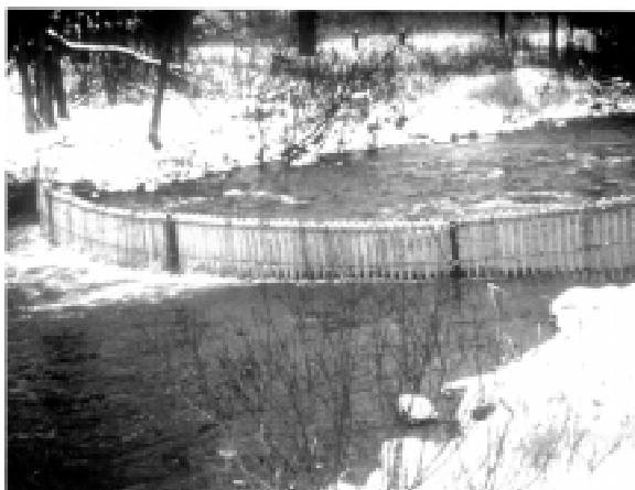
a. Installed condition.
