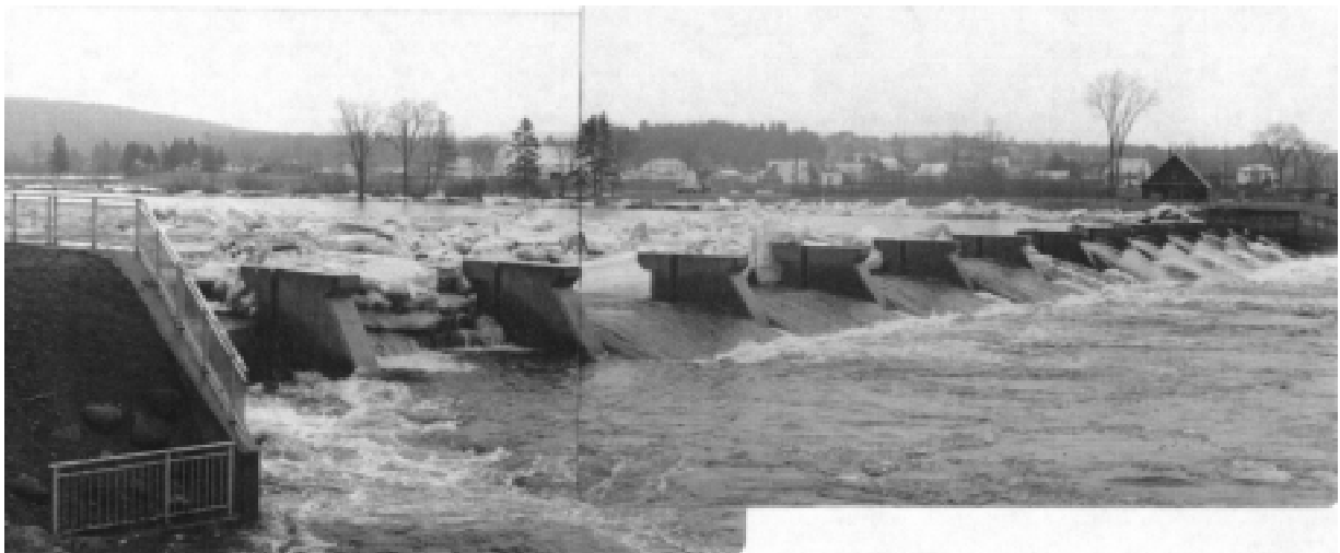
Figure 19. Weir with piers ice control structure on the Ste. Anne River, St. Raymond, Quebec. (Photo courtesy of Marc Delagrave, Roch Itée Groupe-conseil, Sainte-Foy, Quebec.)
