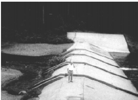
Figure 11. Ice control weir on the Israel River, Lancaster, New Hampshire, July 1994.
