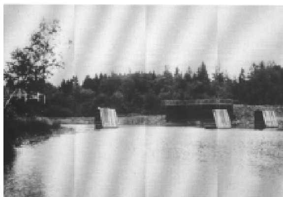
Figure 21. Rock-filled timber cribs upstream of the dam at Cherryfield, Maine.
