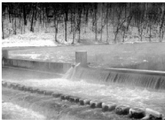
Figure 12. Ice control weir on Oil Creek, upstream of Oil City, Pennsylvania.
