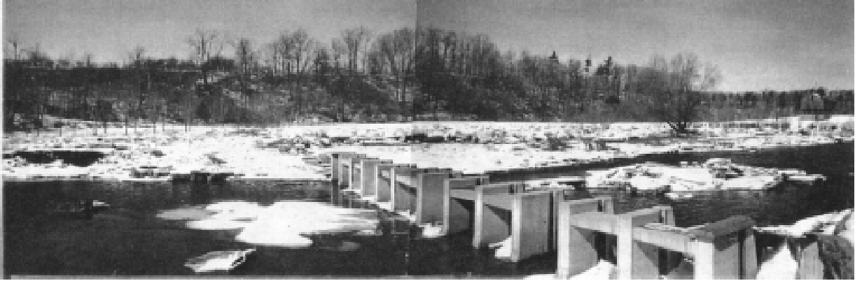
Figure 17. Credit River ice control structure following breakup, March 1994. Note the ice stored on the right flood plain. (Photos courtesy of Harold Belore.)
