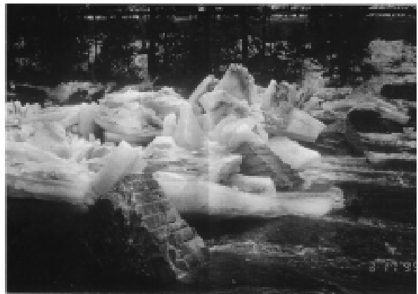
Figure 18. Cut granite block ice control structure in Hardwick, Vermont, following breakup, March 1995.
