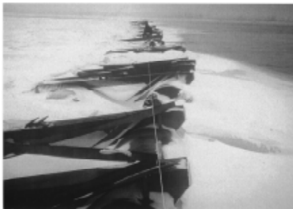
Figure 6. Boom on Beauharnois Canal, constructed of double steel pontoons.
