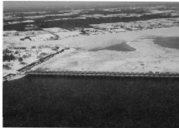
c. Iroquois control structure.
