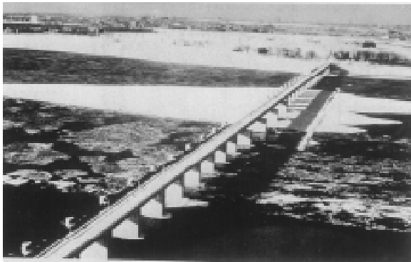
Figure 2. Montreal Harbor ice control structure. (From Lawrie 1972.)
