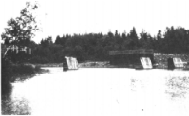
Figure 7. Example of rock-filled crib, Cherryfield, Maine.
