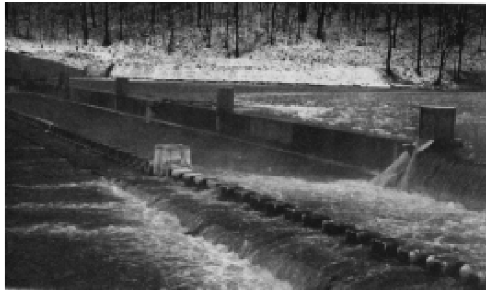
b. Oil Creek ICS in operation.
