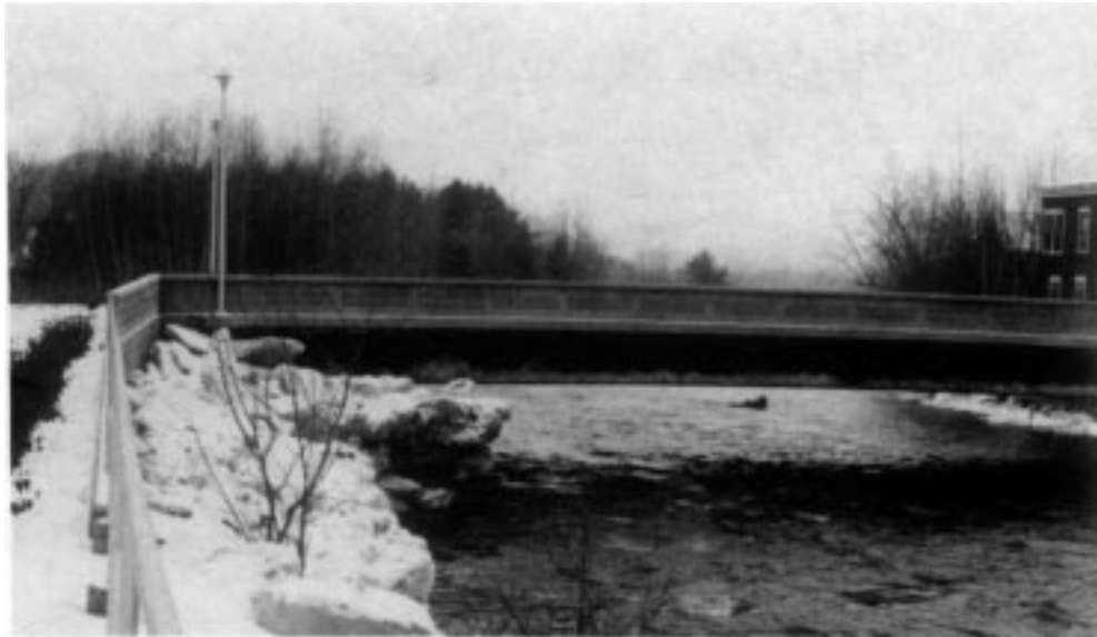
Figure 26. Photographic records can be useful in determining ice jam characteristics. Here ice debris can be seen on the low steel of the bridge, an indication of the ice jam stage. The ice pieces left on the bank indicate that this was a breakup jam that also contained frazil ice (Israel River, N.H.).
