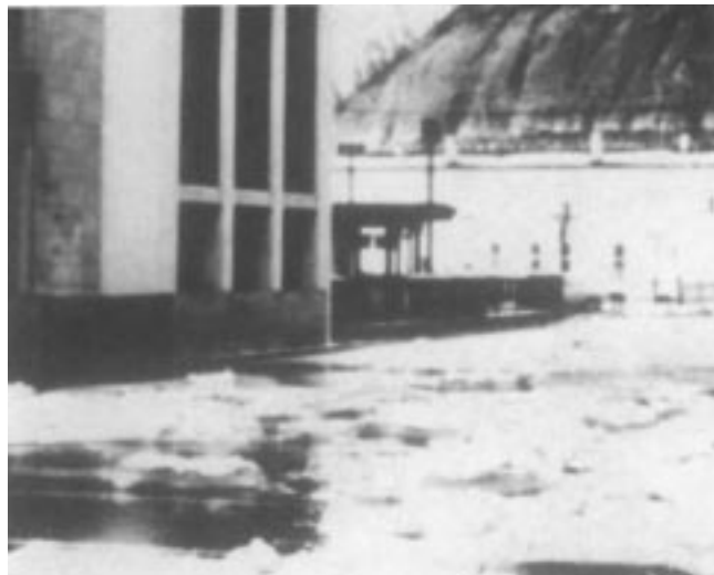
b. Looking across street to the same location, after flooding.
