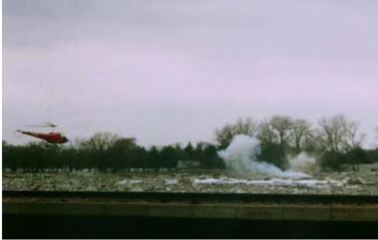
Figure 4. Blasting on the Platte River near Ashland in February 1997. Following a devastating jam in 1993, state and Federal officials developed a rapid response plan that allows blasting to begin within hours. (Photo courtesy of J. Mastandrea, Sarpy County, Nebraska, Emergency Management Agency.)
