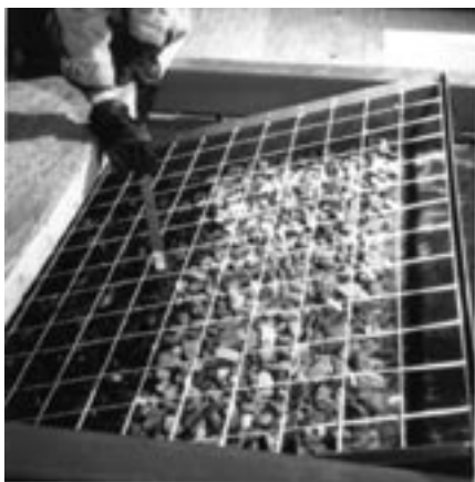
Figure 13. Measurement of the distance of the riprap surface from the strings at each grid point.
