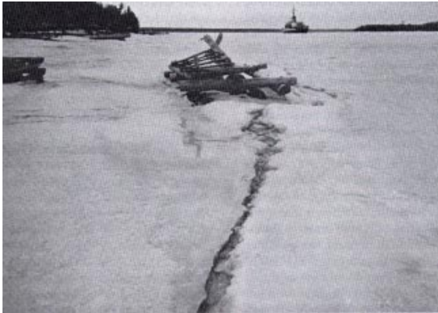
Figure 13. Active crack passing through a damaged dock.
