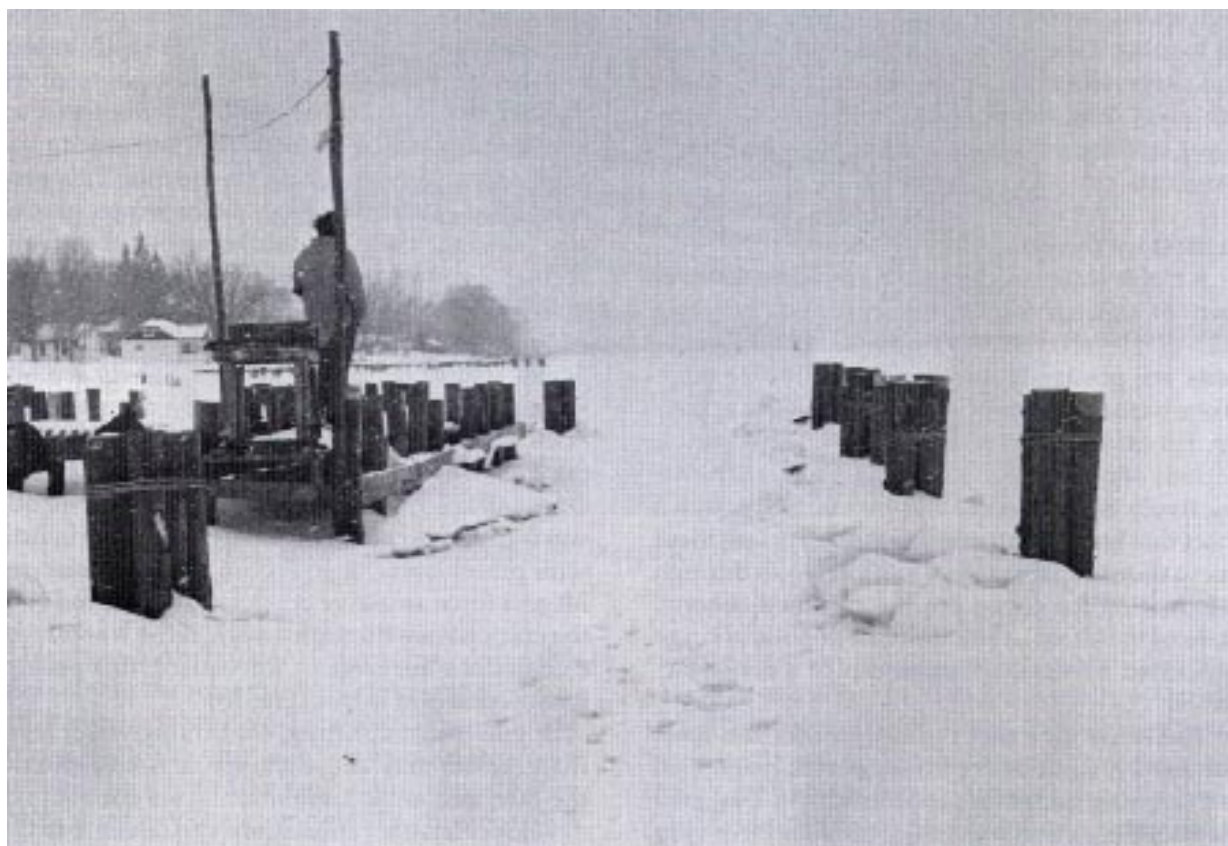
Figure 12. Private dock on the St. Marys River with protective pile clusters.
