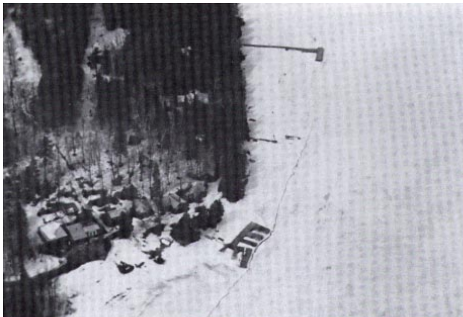
Figure 11. Aerial view of Johnson's Point, showing active crack offshore of structures.
