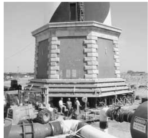
The lighthouse tower on a temporary support system. Note one of a series of sensors (at right on tower base) which will be connected to a central monitor to direct the operator to adjust the hydraulic jacks that will support the tower during the move. Photo by Steve Kozosky.
