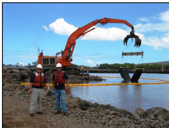
Ongoing Harbor Construction at Kikiaola Small Boat Harbor
