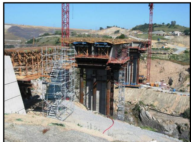
On-going construction at Folsom Bridge
