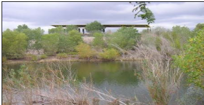
Completed section of Rio Salado project with environmental measures.
