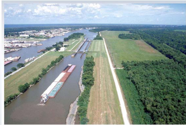
Bayou Boeuf Lock, Louisiana. Courtesy of USACE Digital Image Library
