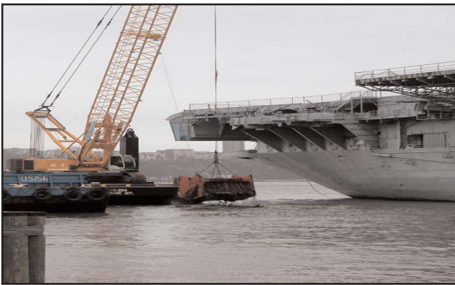
Ongoing Dredging operations alongside the USS Intrepid.
