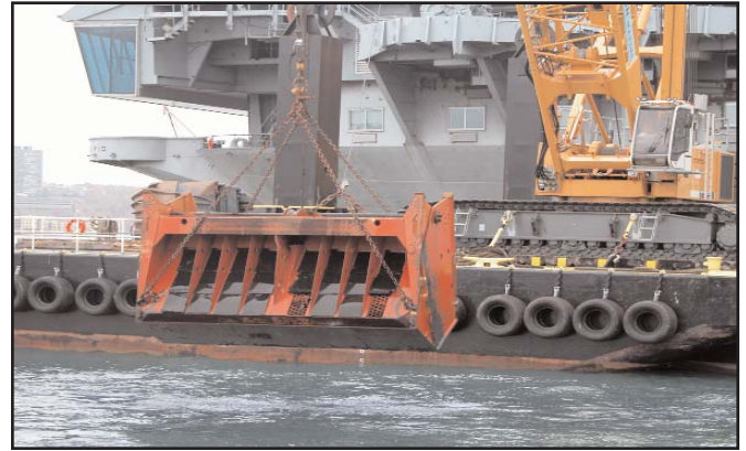
Ongoing Dredging operations alongside the USS Intrepid.
