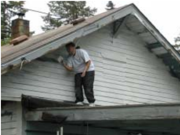
Becky Dansereau helps paint the roof.
