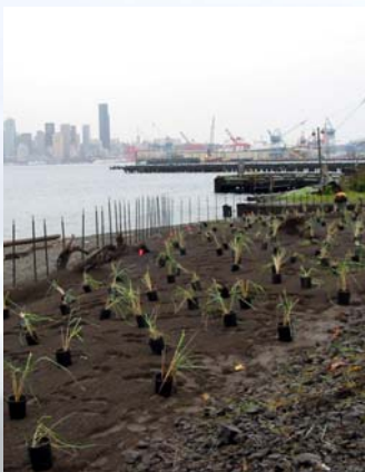
Cover: Crews plant native beach grass at the east end of the Pacific Sound Resources shore site. (Cover: file photo; Col. Lewis, Seattle skyline and watermark are file photos)
