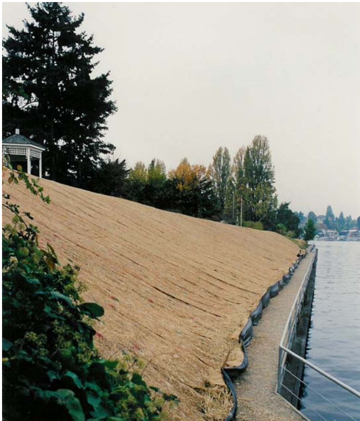
Re-graded and stabilized bank—after.
