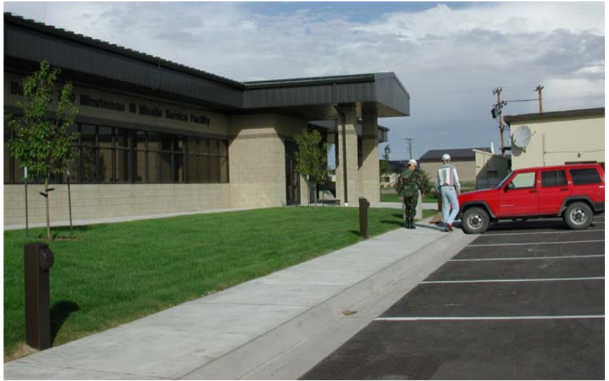
Minuteman missile service facility at Malmstrom Air Force Base, Mont.
