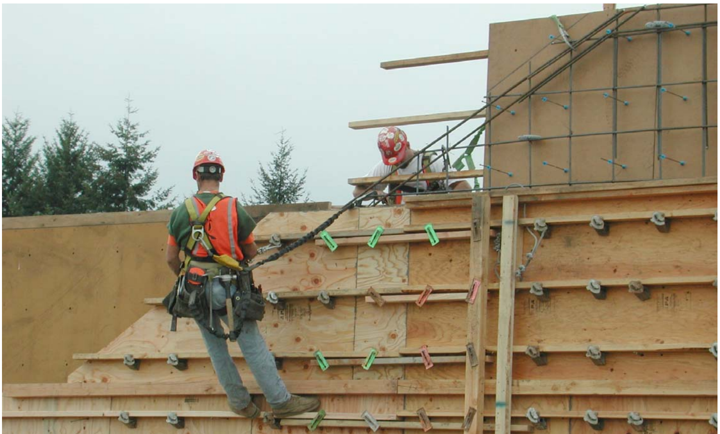
“On rappel!”—Formworkers prepare the walls for concrete on the 300-person barracks.
