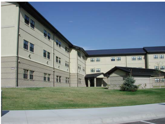
The 741st Security Forces Squadron dormitory, constructed by the Corps at Malmstrom AFB.
