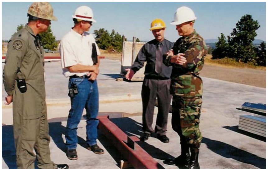
Project Manager Andy Maser explains the JPRA project to Col. Graves.
