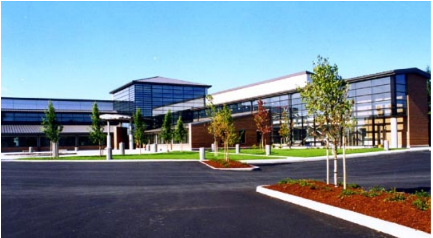
The front entrance of the 90,000-square-foot medical clinic.
