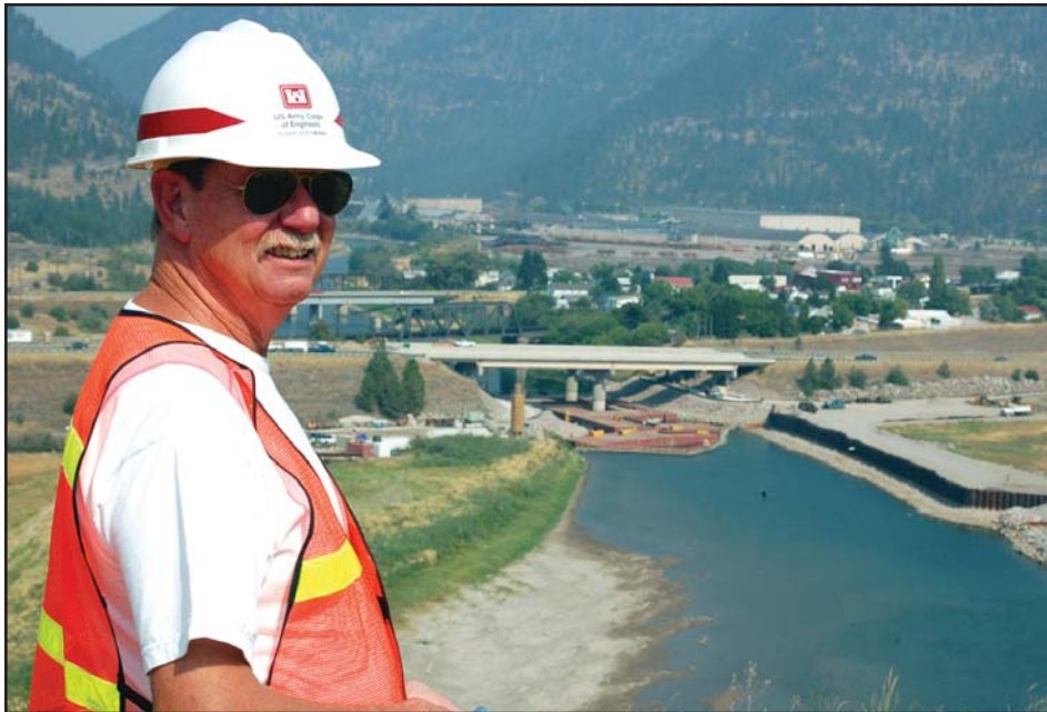
Terry Hoffman, the projects' Quality Assurance inspector and retired annuitant, describes the view from "the overlook" above the Milltown Dam. Clearly visible are the Blackfoot River (to the left) the I-90 bridges (center) and the sheet pile wall and bypass channel under construction. Out of the frame to the right is the Clark Fork River. (Dick Devlin Photo) OPPOSITE PAGE: Corps engineers watch from above as the river begins to run freely following the removal of the coffer dam. (Sara Malo Photo)
