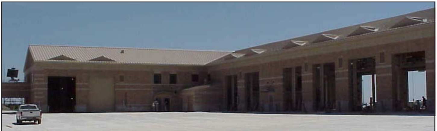
The 726 Air Control Squadron complex contains a new vehicle maintenance building, shown here, which will allow for maintenance of the fleet and satellite communication system as well as new office space. Photo provided by Mark Slominski
