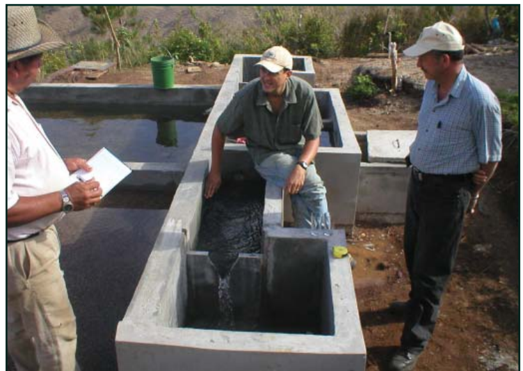
Owen Reese (sitting) explains to the two Hondurans who will operate it, a multi-phase slow sand filter he and his wife, Amy Reese, built for the community of Los Arcos. This is the slow sand filter. Not pictured is the coarse up-flow filter. These filters remove 99.99% of parasites and the majority of bacteria, the rest of which are removed by the chlorine addition down at the storage tank. (Amy Reese Photos)
