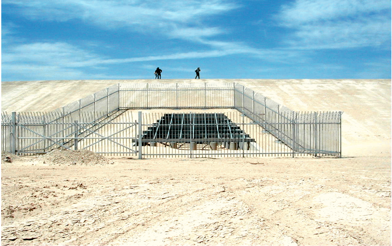
Photo 3. Tropicana Detention Basin . Outlet works intake structure.
