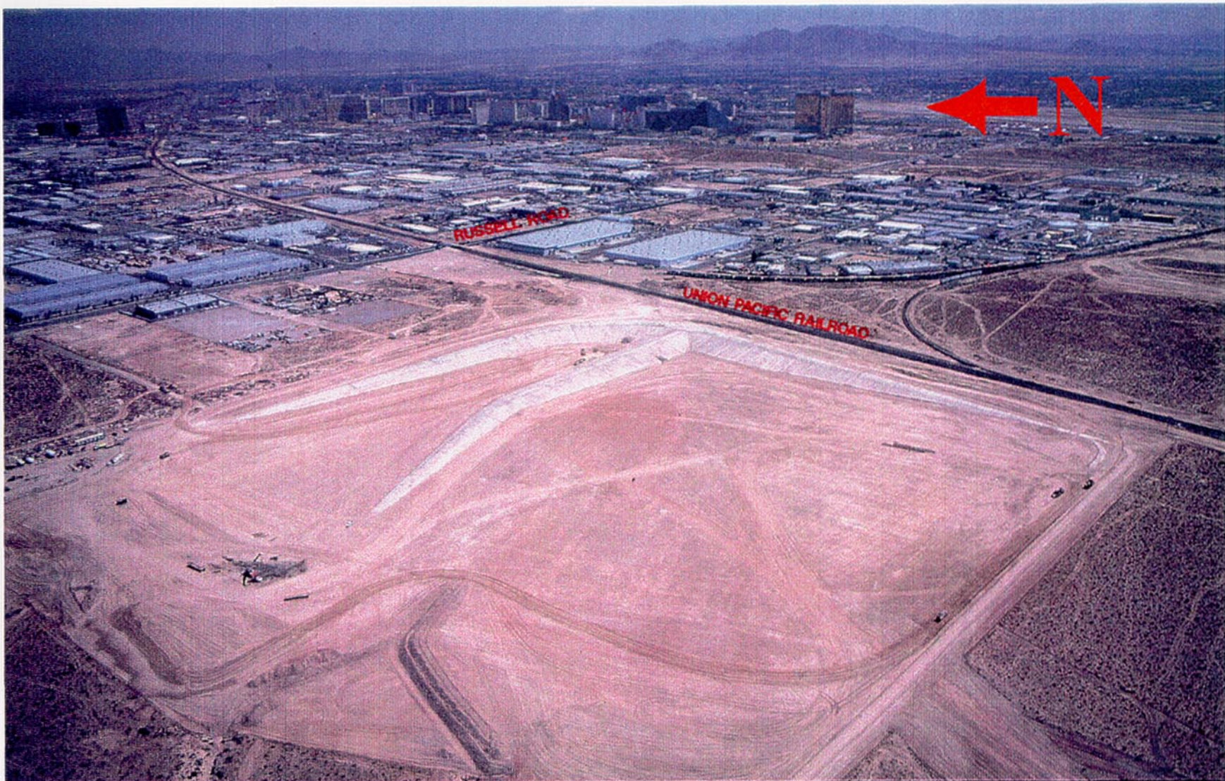
Tropicana Detention Basin - 15 May 1998
