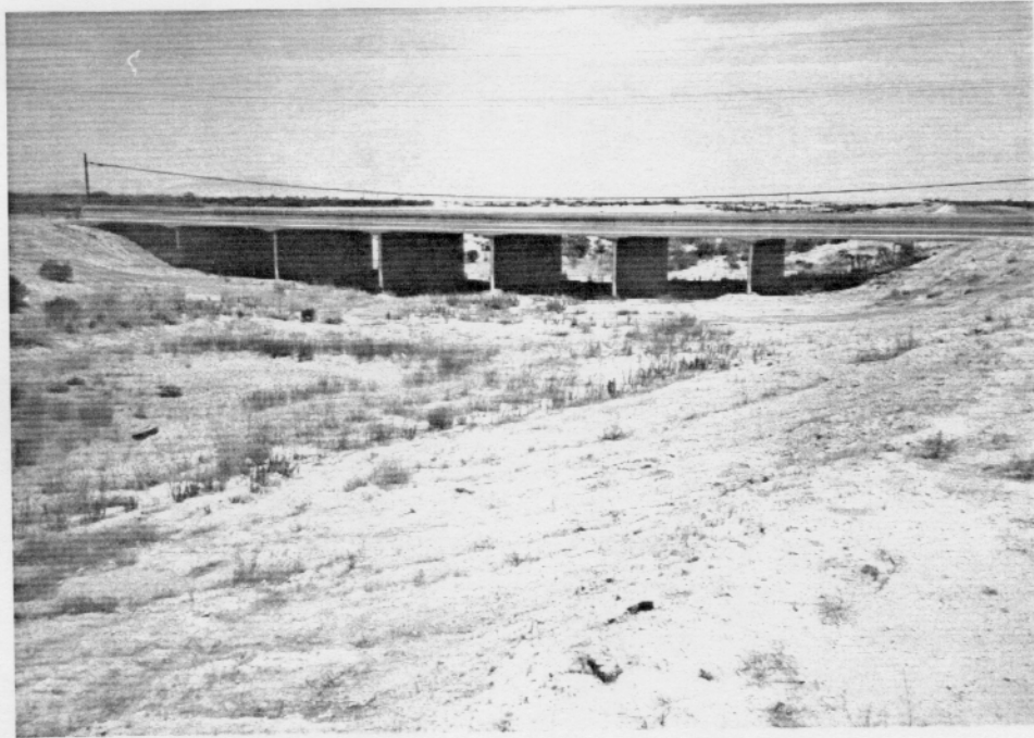
Photo 3-02. Bridge crossing over channelized section of Santa Rosa Wash approximately 17 miles downstream of the dam (looking downstream).
