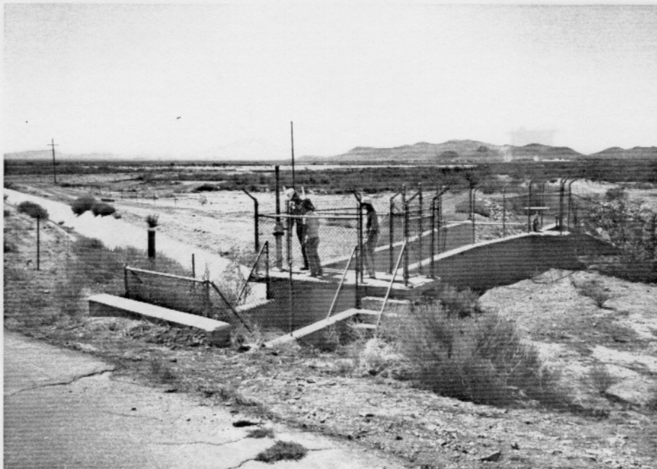
Photo 2-08. Conservation Outlet Works Stilling Basin and Vaiva Vo Irrigation Project Canal (background left; looking northwest from the road).
