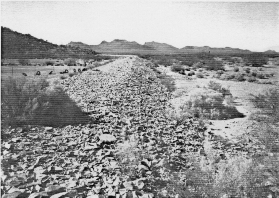
Photo 2-04. Tat Momolikot Village Dike (looking north along the east village dike).
