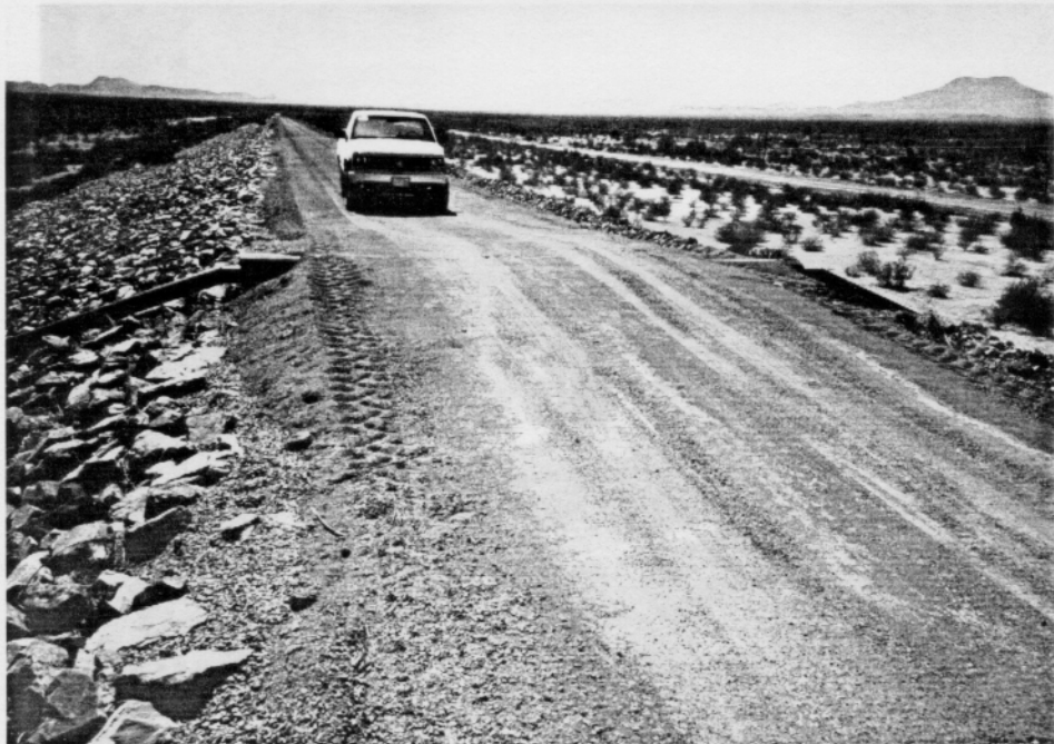
Photo No. 2-01. Pipeline Crossing over Dam Embankment.
