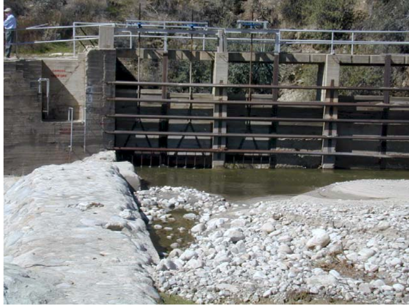
Photo 3-1. Upstream View of SBVWCD Diversion Structure
