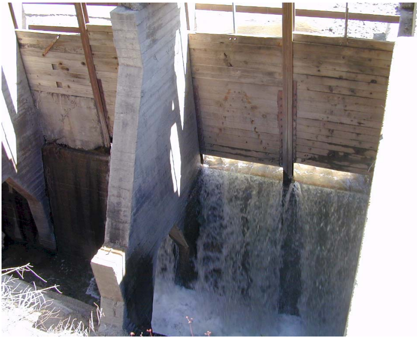
Photo 3-2. Downstream View of SBVWCD Diversion Structure
