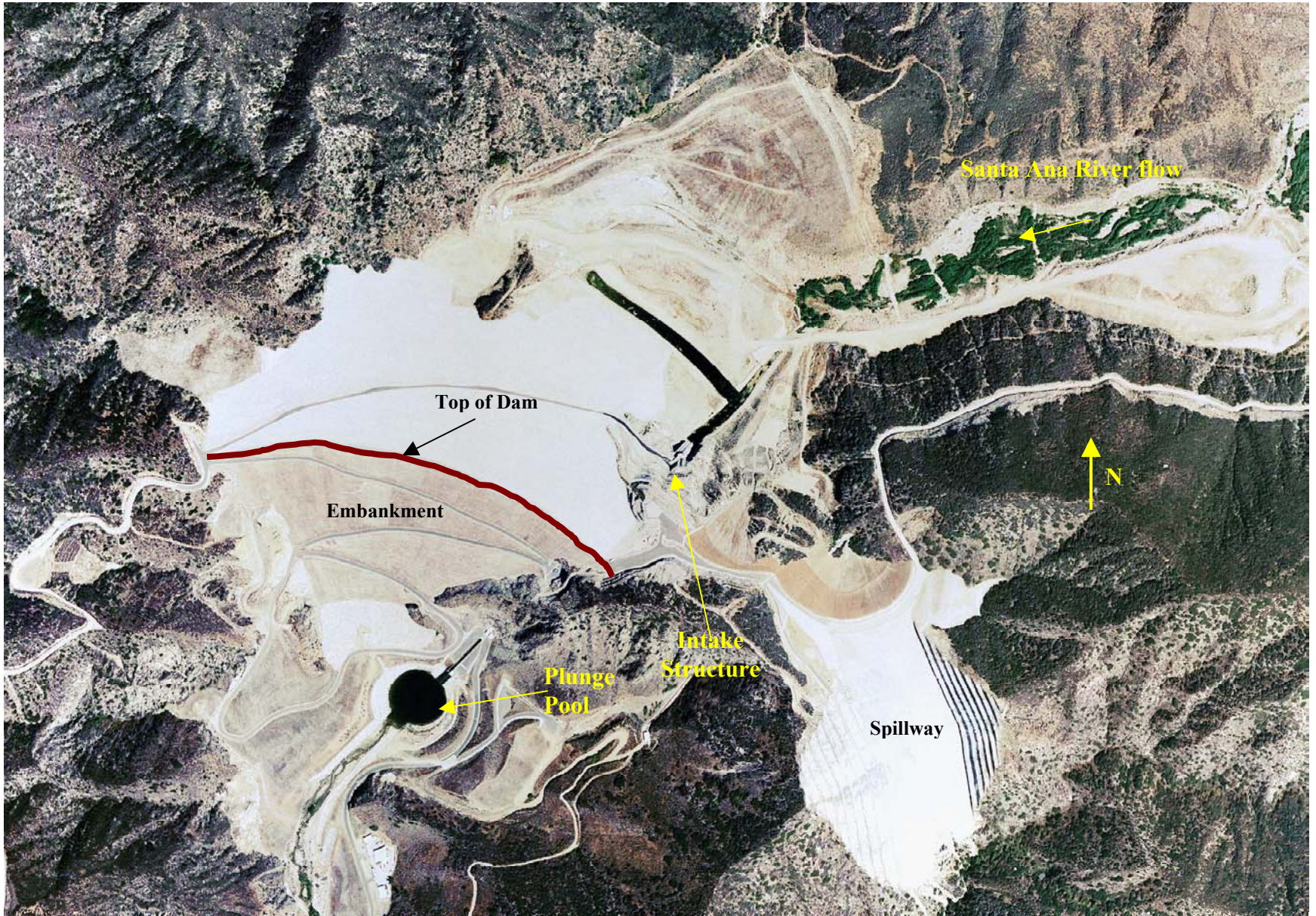
Aerial Photograph of Seven Oaks Dam and Reservoir
