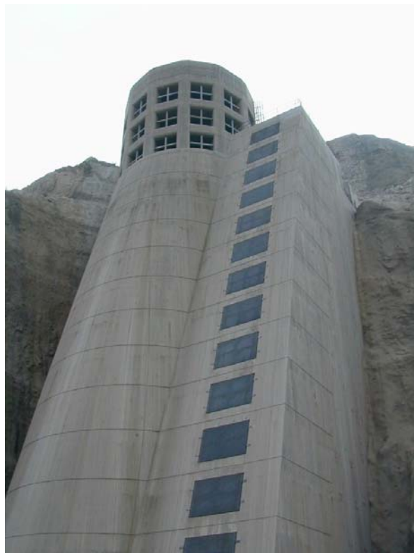
Photo 2-3. Intake Tower - MLS (on left) and MWS (on right)
