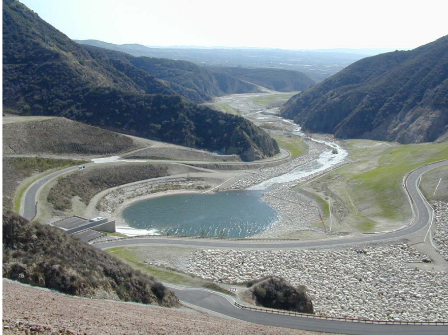
Photo 2-6. Looking Downstream at the Plunge Pool from Top of Embankment
