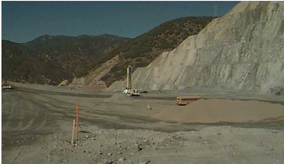
Photo 2-8. Looking Upstream During Spillway Excavation
