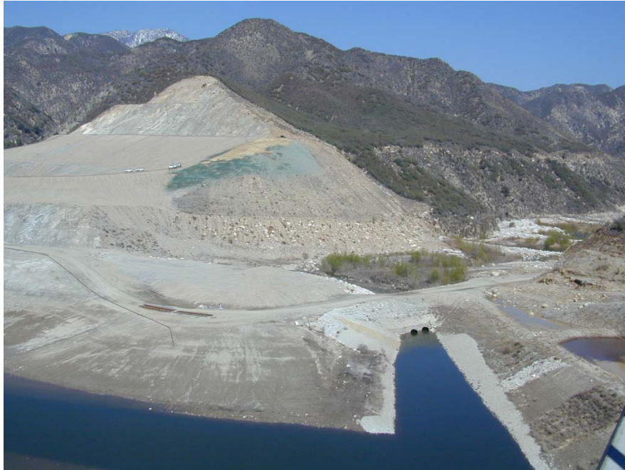
Photo 2-2. Looking Upstream from Top of Intake Tower towards Government Canyon Ridge
