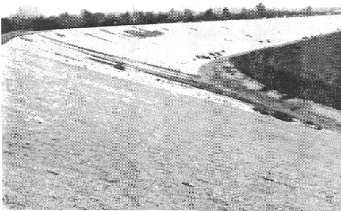
Photo No. 2-09. Upstream Slope of Dam Northeast of Spillway (view toward south, from east embankment of dam.)
