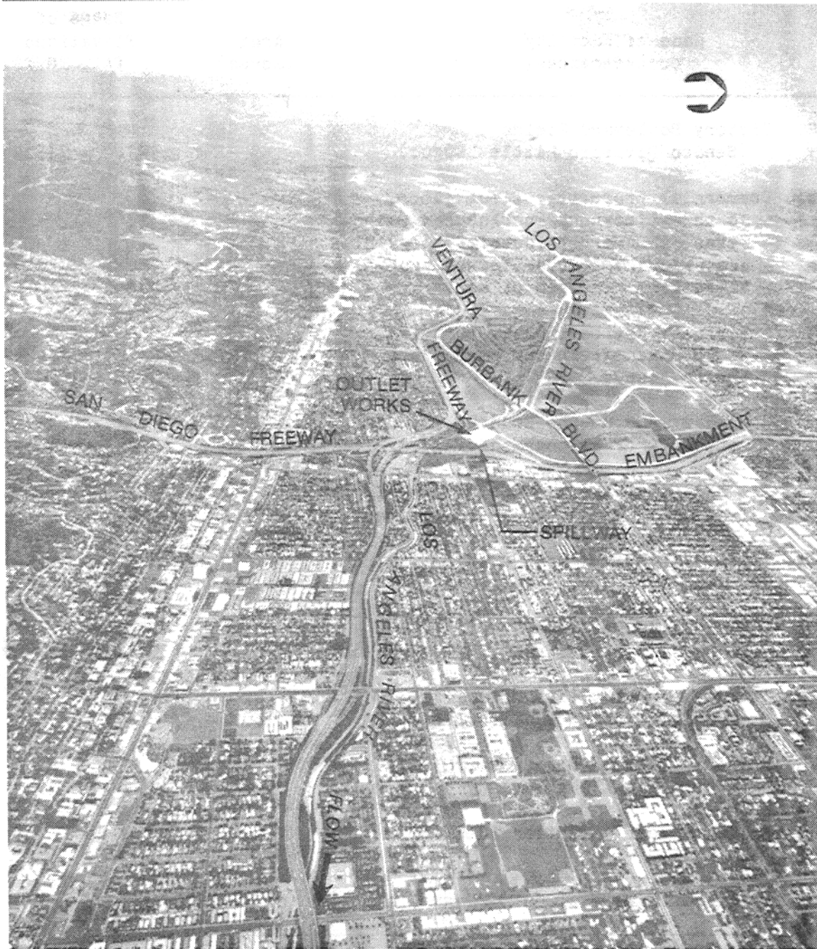
Photo No. 2-01. Los Angeles River, with Sepulveda Dam and Reservoir (view from downstream of dam, taken 5/6/75).
