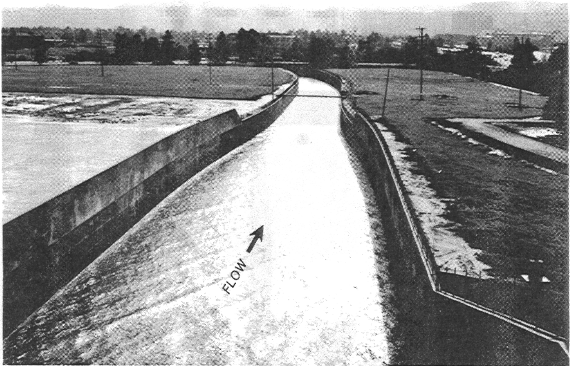
Photo No. 2-17. Los Angeles River: Outlet Channel, with Spillway Apron on left (view toward downstream from bridge above outlet works during high outflows of February 1980).
