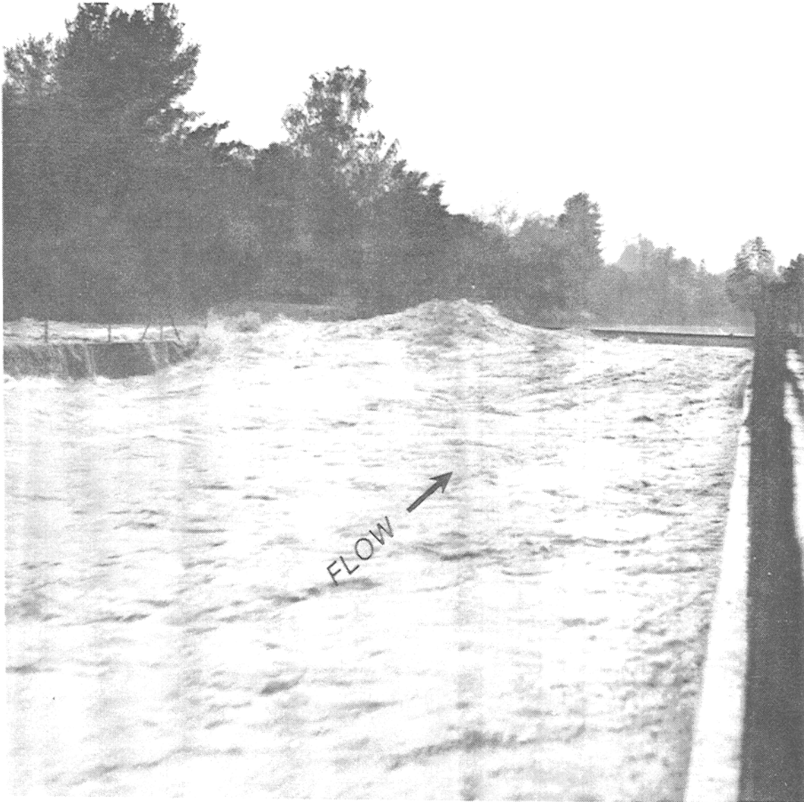
Photo No. 4-01. Flood of 16 February 1980, Los Angeles River at Cedros Street, approximately 1.5 river miles below Sepulveda Dam (view toward downstream, showing overflow of left bank resulting from hydraulic instability due to a side drain in the channel wall).
