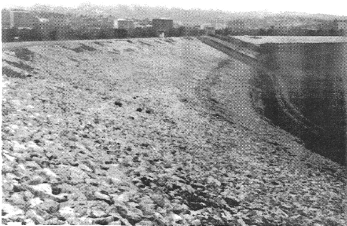
Photo No. 2-07. Upstream Slope of Dam Southwest of Outlet Works (view toward southwest, from outlet works).
