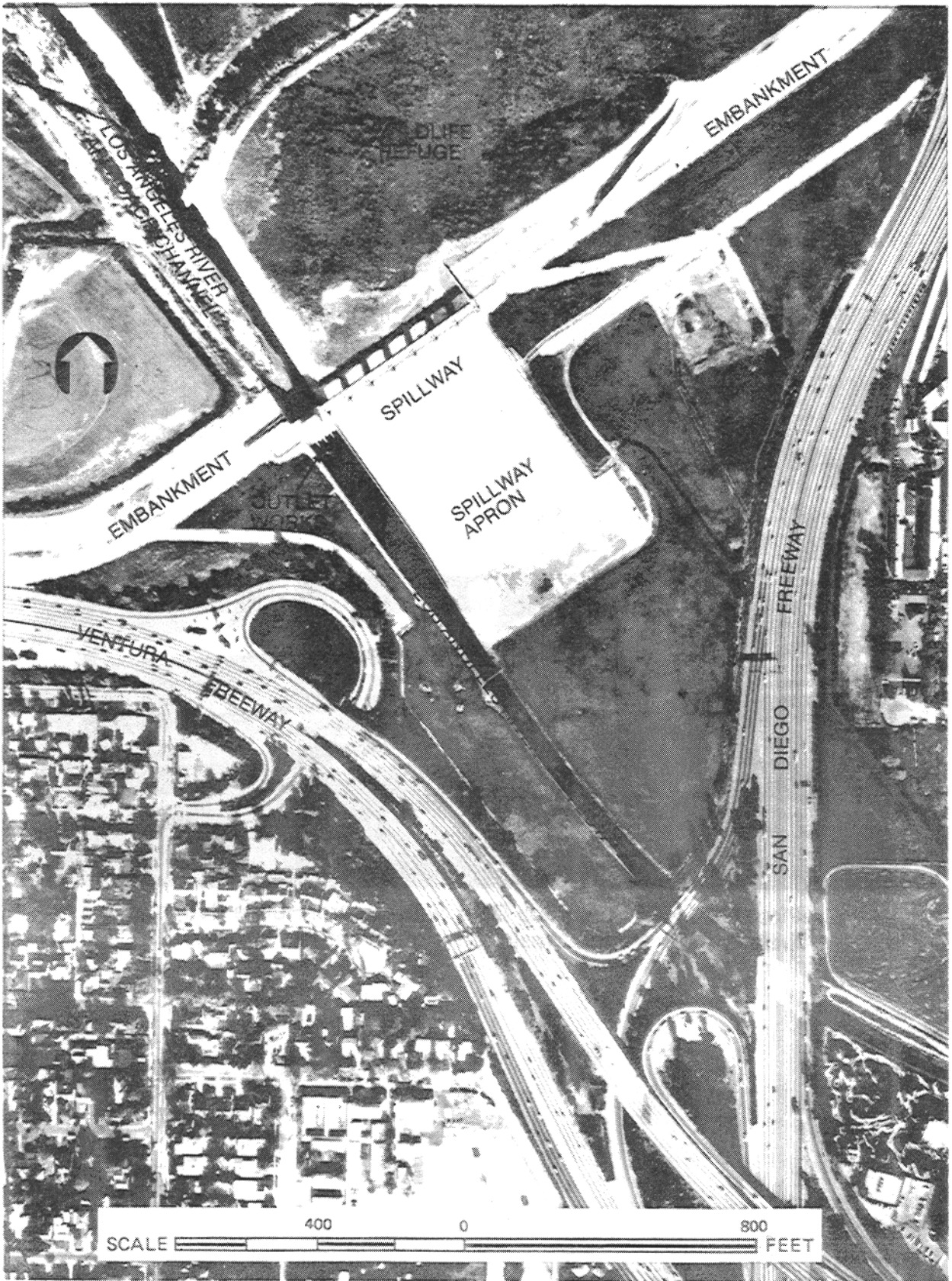
Photo No. 2-04. Sepulveda Dam (enlargement of Photo No. 2-03).
