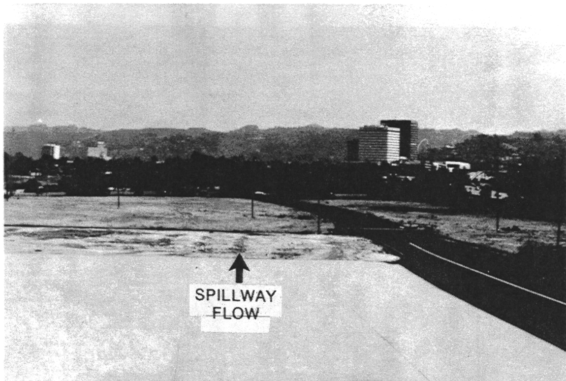
Photo No. 2-23. Spillway Apron, with Outlet Channel to right (view from spillway bridge, toward downstream).
