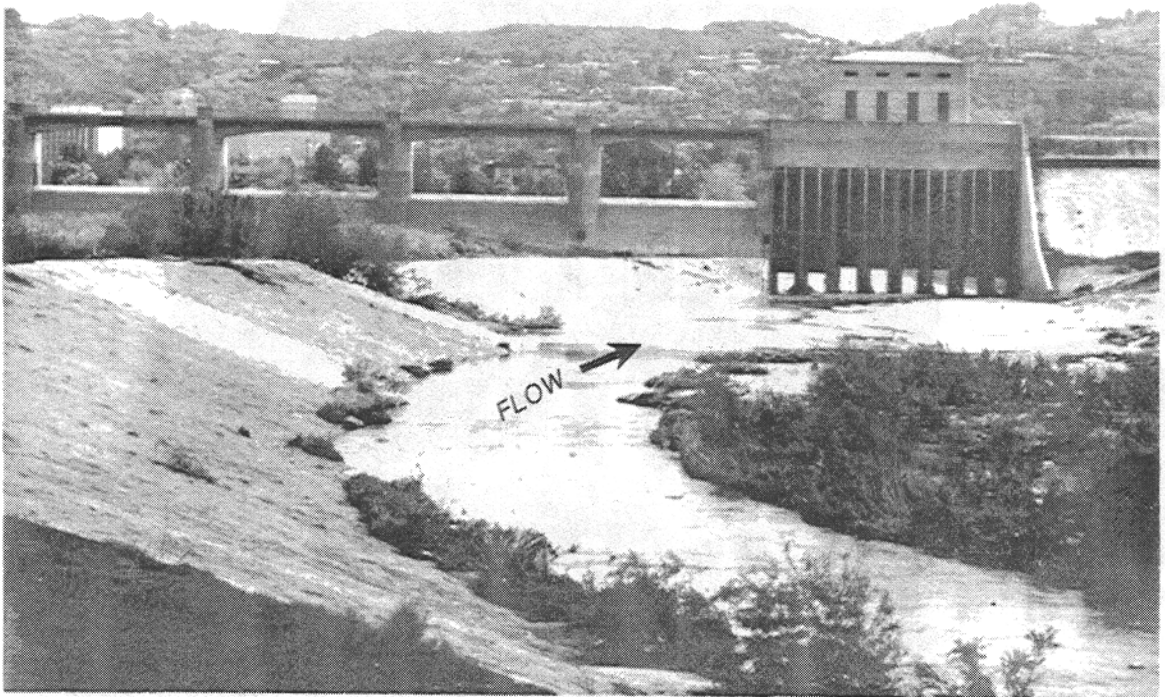
Photo No. 2-11. Control House and Outlet Works, with Spillway to left (view from upstream, within reservoir, along approach channel)
