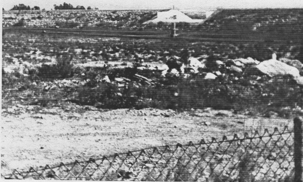
Figure 3-02 Cucamonga Canyon Debris Basin. Looking Southeast.
