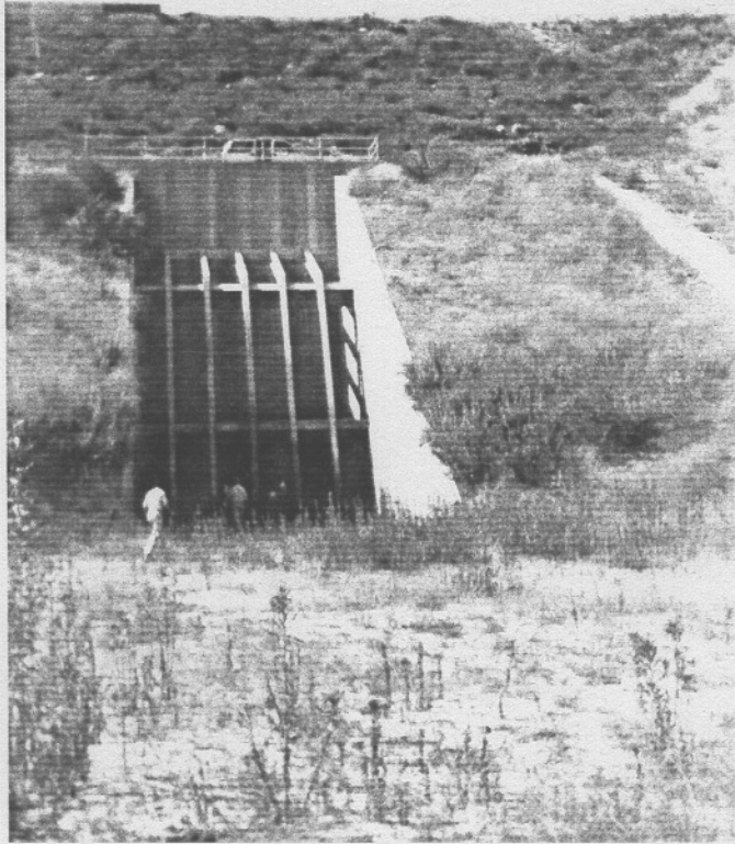
Figure 2-02 Outlet works at San Antonio Dam. Elevation 2125 ft. NGVD. Control House at top of Dam. Looking South.
