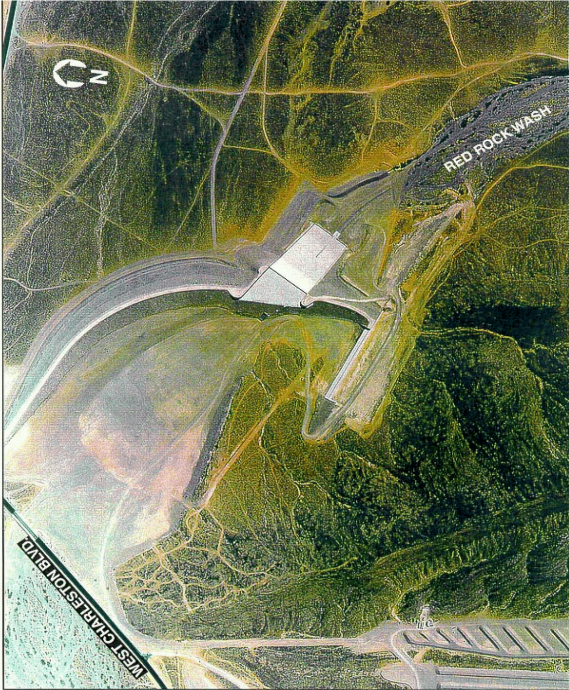
Red Rock Detention Basin - 13 April 1997
