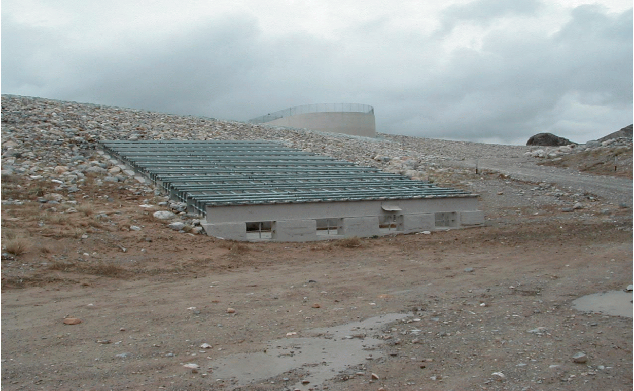
Photo 3. Red Rock Detention Basin . Outlet works trashrack.
