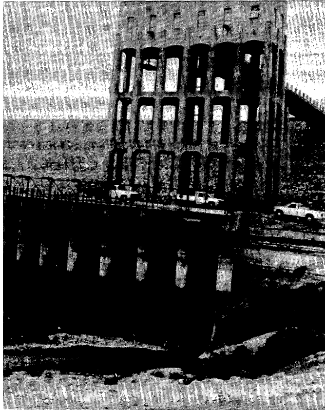
Photo 2-2: Prado Dam - View of the approach channel and intake structure
