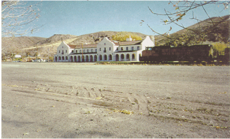
Photo 2-1. Union Pacific Railroad at Caliente, Nevada.
