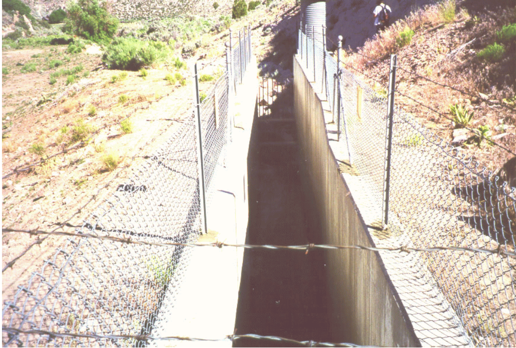
Photo 2-5. Looking downstream at stilling basin.
