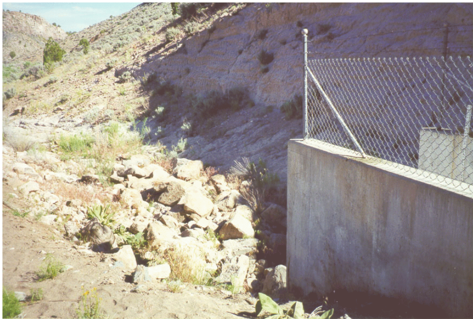
Photo 2-6. Riprap at the Transition from Stilling Basin to Outlet Channel
