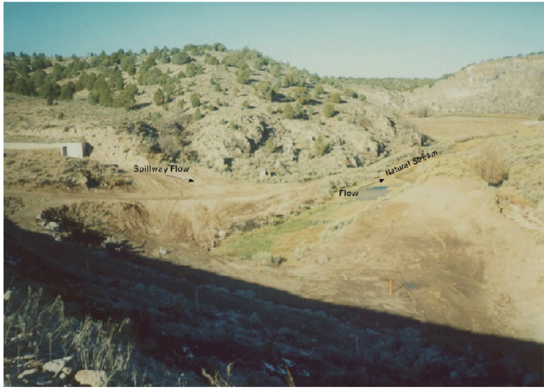
Photo 4-1. Looking downstream below spillway
