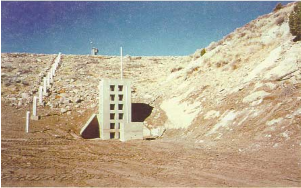
Photo 2-3. Intake structure and staff boards at right abutment.
