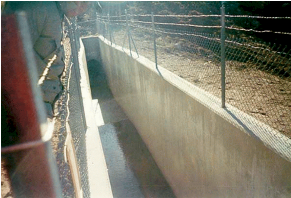
Photo 2-4. Looking upstream at outlet tunnel and stilling basin.
