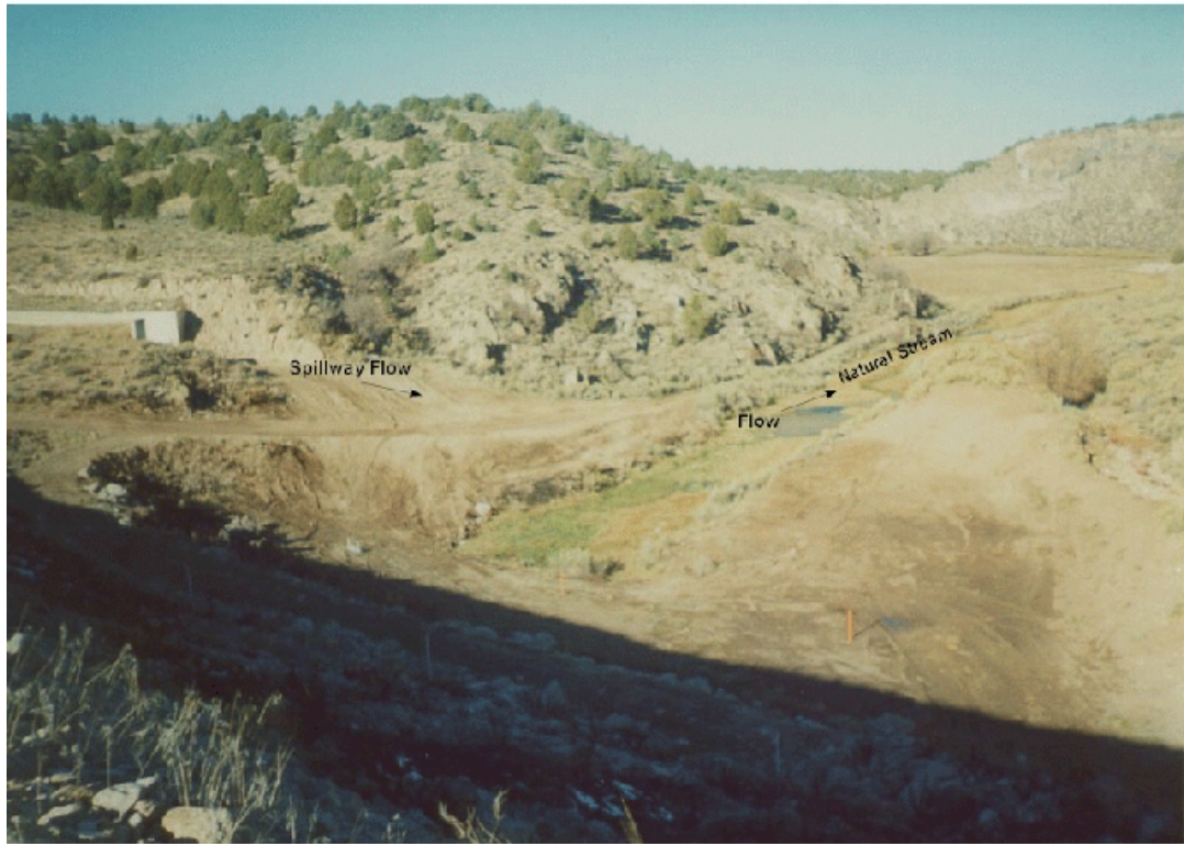
Photo 4-1. Looking downstream below spillway
