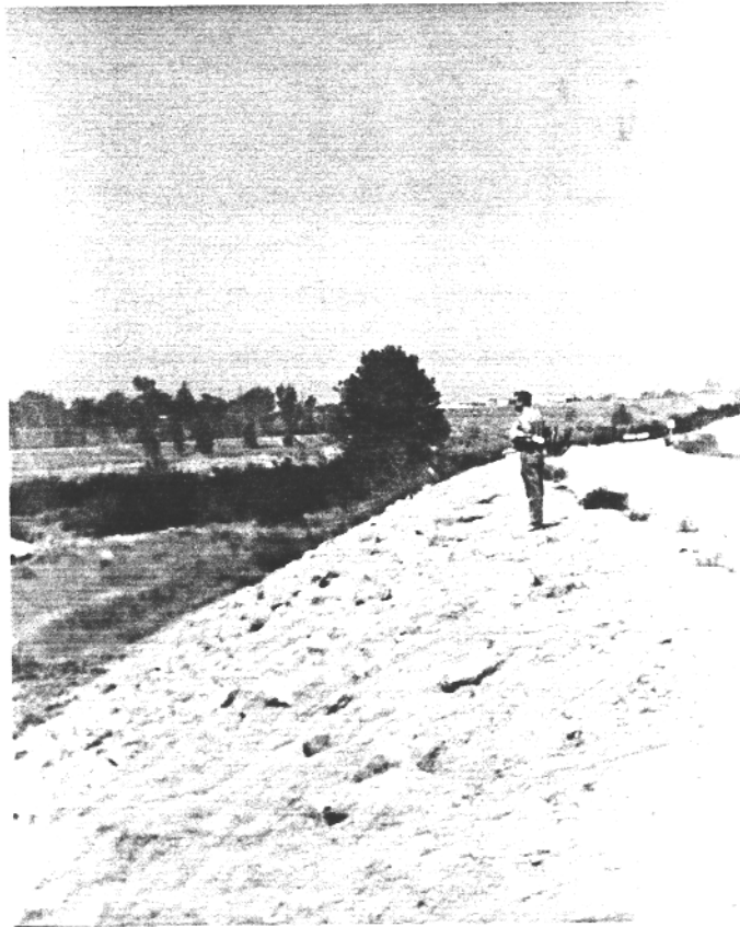
Figure 19. Looking NW Along Grouted Quarry Stone Of Muscoy Levee Near The Junction Of East Side Of Lytle Creek Intake Structure With Muscoy Levee.
