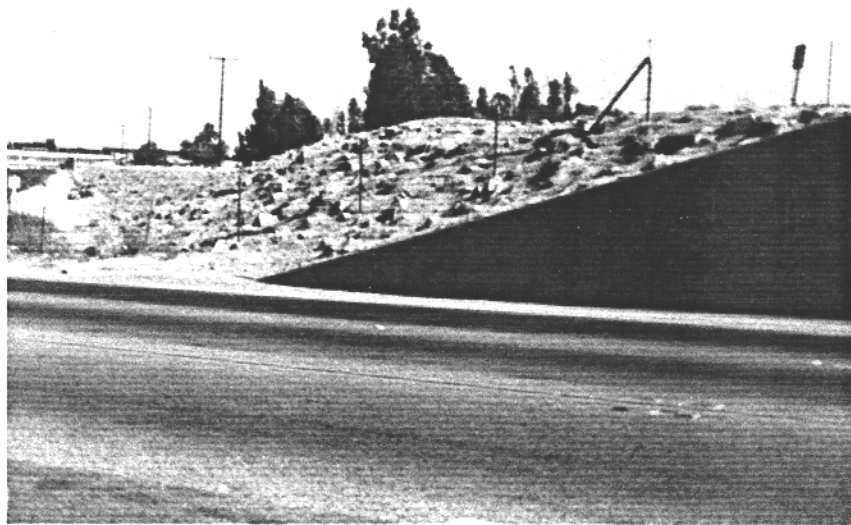
Figure 26. Grouted Quarry Stone Of Island Levee At Highland Avenue Looking South On Lytle-Cajon Drainage, San Bernardino County, California.
