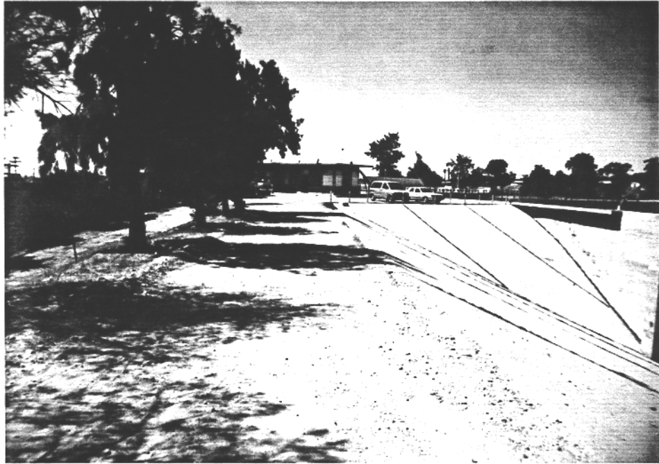
Figure 3. Lytle Creek Intake Structure Looking SW At Control House At West Branch Intake. East Wing Levee In Background.
