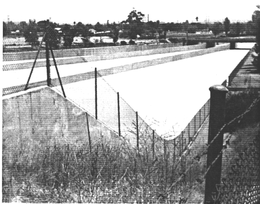
Figure 14. East Branch Lytle Creek Channel Looking SE. The 58,000 c.f.s. Capacity Channel Is 400 Feet Wide With Training Walls At 132 Foot Intervals.
