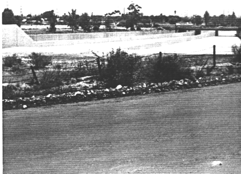
Figure 16. Looking SE Along Lytle Creek East Branch Channel. Flows Above 22,800 c.f.s. Will Begin To Flow Around The Left Wing Levee And A Portion Will Begin To Flow Down The East Branch Channel.
